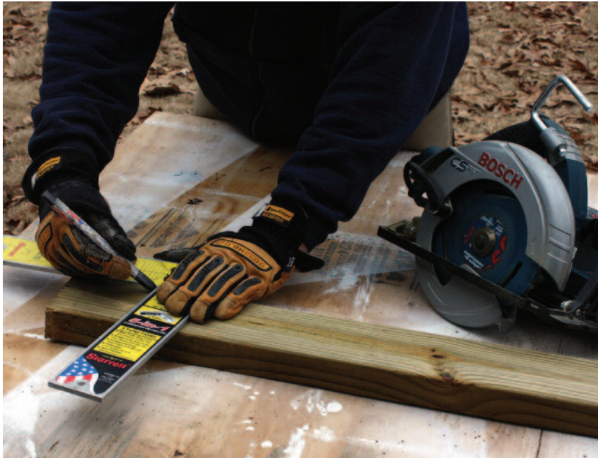
If you're toe-nailing the fence, then the stringers that follow a slope should be cut at a miter to fit flush between the plumb posts.
