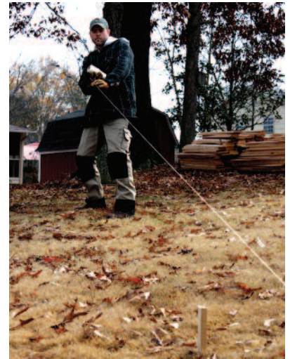
With the line in place, measure for the fence post locations and spray paint an "X" over the exact spot to dig.
