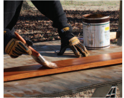
I used Armstrong-Clark's semi-transparent Sierra Redwood stain, and highly recommend applying it to the materials prior to assembly. It's much easier.
