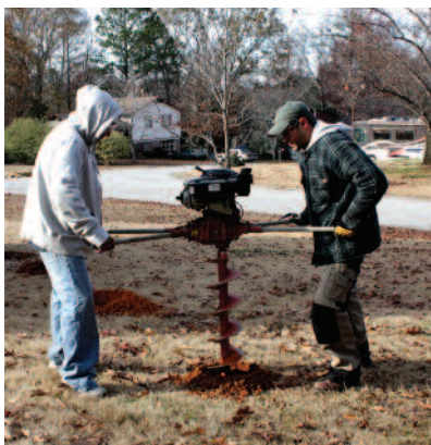
A rented two-man power auger and an electric demolition hammer helped greatly when digging the holes.
