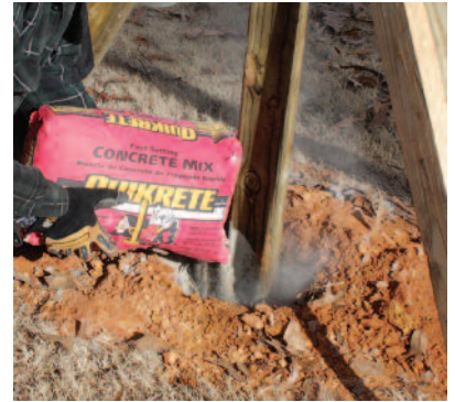
Quikrete Fast-Setting Concrete can be easily poured into the post hole dry. No mixing is required.
