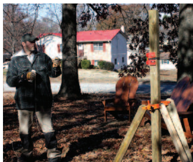
Set the corner posts first, stringing a new line between to line up the other posts.
