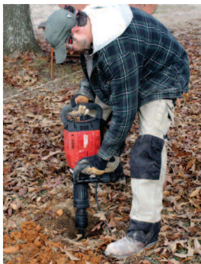
A rented two-man power auger and an electric demolition hammer helped greatly when digging the holes.
