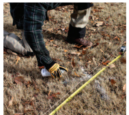
With the line in place, measure for the fence post locations and spray paint an "X" over the exact spot to dig.
