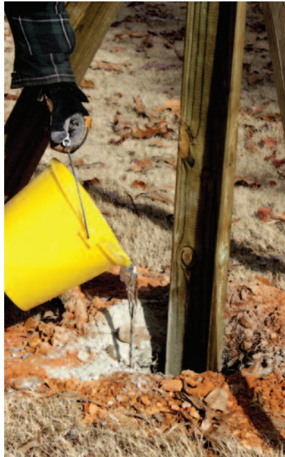
Pour the water over the dry concrete to set the posts.
