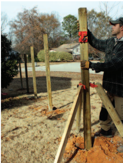
A Post-Pod ( cepcotool.com ) is helpful for one-man installation.
