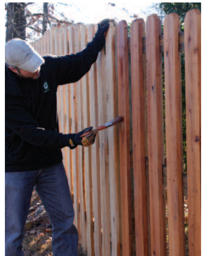
I used Armstrong-Clark's semi-transparent Sierra Redwood stain, and highly recommend applying it to the materials prior to assembly. It's much easier.
