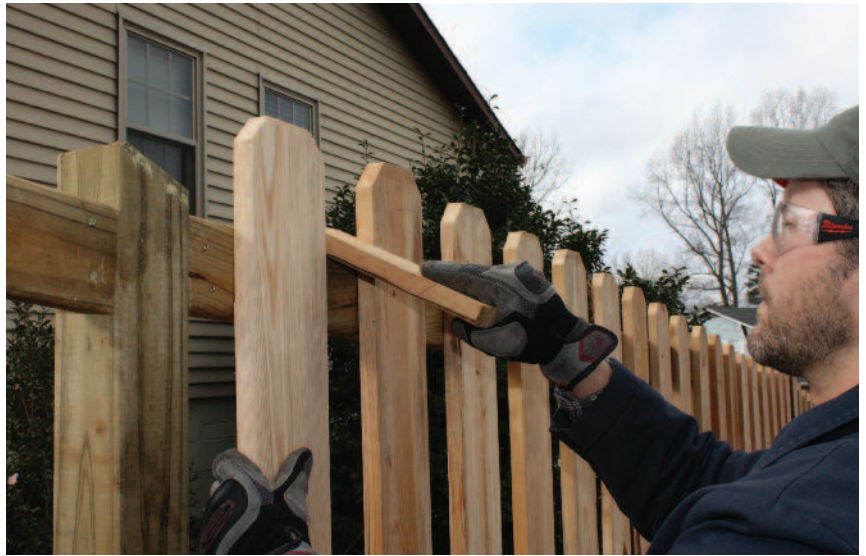
I used a homemade spacing block to keep the pickets even.
