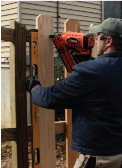
Drive two nails through the fence board at each stringer location.
